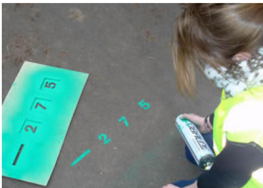
Markings along the river for 20ft to an Inch
